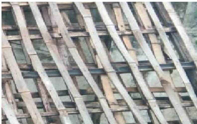
Fig 2: Bamboo Strips Reinforcement for Slab
