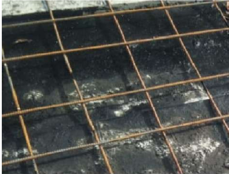
Fig 1: Steel Bar Reinforcement For Slab
