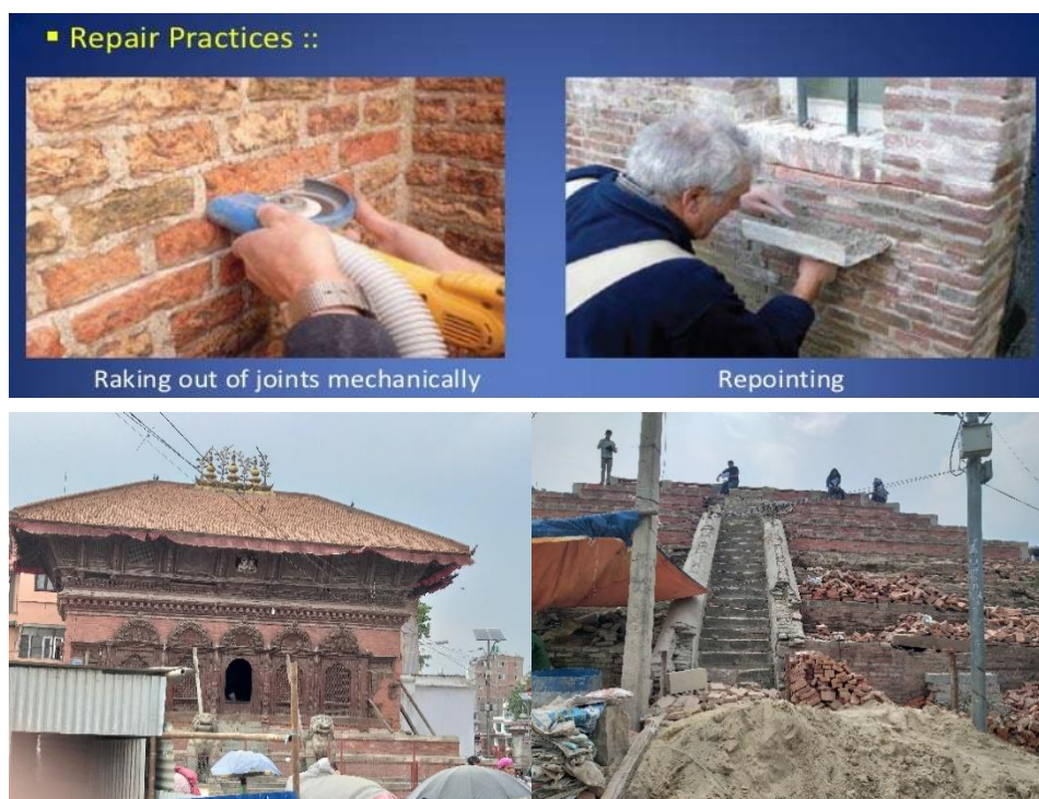
Figure 7 Image showing repair remedial practices over heritage assemblies Source: Photographs clicked by authors during the site survey, Nepal.
