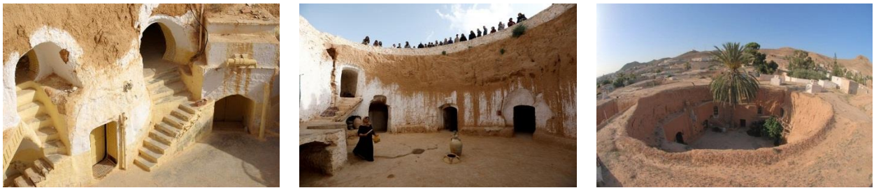
Figure 7. Underground houses in Matmata, Deep central courtyards (Crouch & Johnson, 2001)
